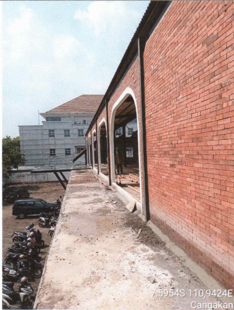
100 % DINDING EXPOSE LANTAI 2
